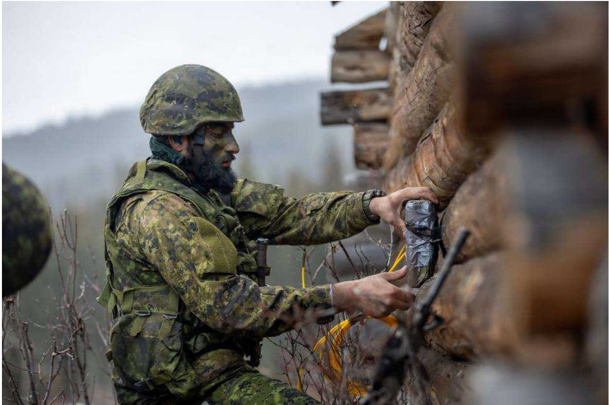
Engineers of The 39 Combat Engineer Regiment place explosive charges at the demolition range during the penetration demonstration (PENDEM) Range
