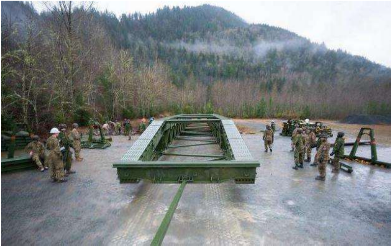
A POV from the driver of an HLWV as they boom a nearly completed MGB across the gap.
