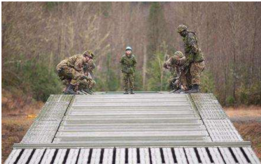
MCpl Au (CJOC), MGB Stand OPT looks on as the decking units are placed on the second MGB build of the exercise.
