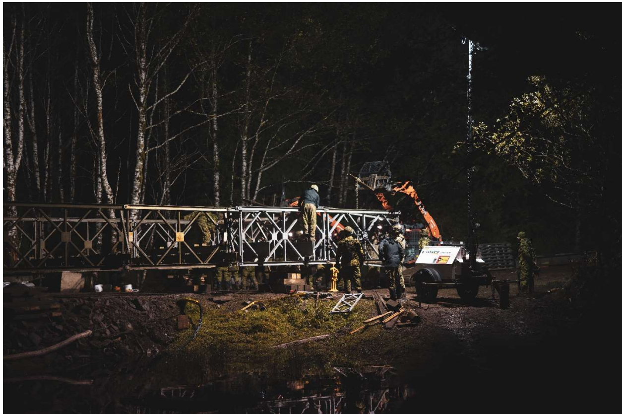
Ex HS 21 – Photo 3: Members of 39 Combat Engineer Regiment construct a permanent ACROW bridge for Canadian Forces Detachment Masset, in Masset British Columbia. 24 September 2021. Photo: Private Daniel Pereira, 39 CBG Public Affairs
