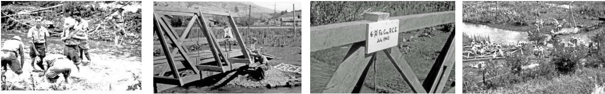
Timber Bridge constructed by 6 Fd Coy R.C.E. Reserves in the summer of 1942 (6FESMA)
