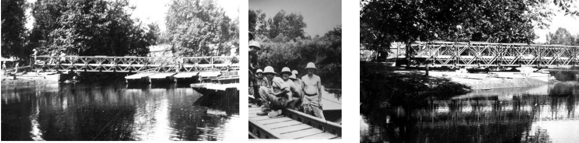
Floating Bailey Bridge constructed by 6 Fd Coy R.C.E. Reserves in 1945 (6FESMA)
