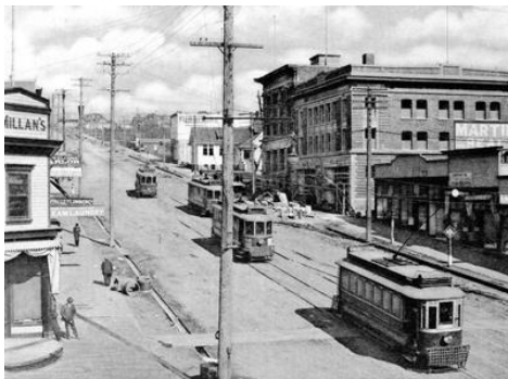
Lonsdale Avenue in North Vancouver 1910 (NVMA)
