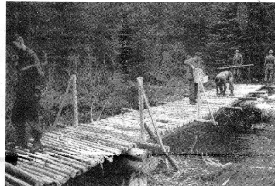
BRIDGE construction — Nancy Greene / Blueberry Paulson area.
