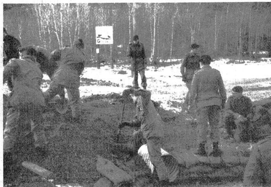
ROAD construction at the Casino Range.
